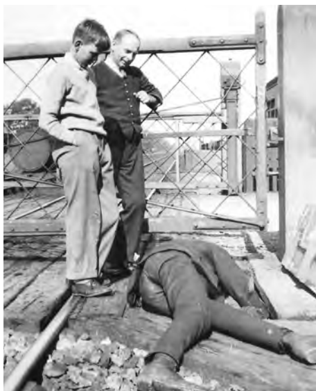
Oiling the level crossing gate near Barnby Moor and Sutton station on the East Coast Main Line. David Maltby looks on as one of the railwaymen explains the procedure.
